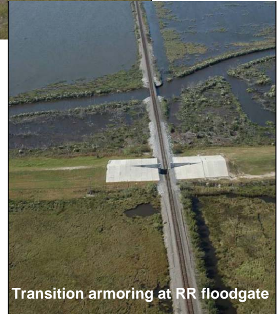
Concrete slope paving
